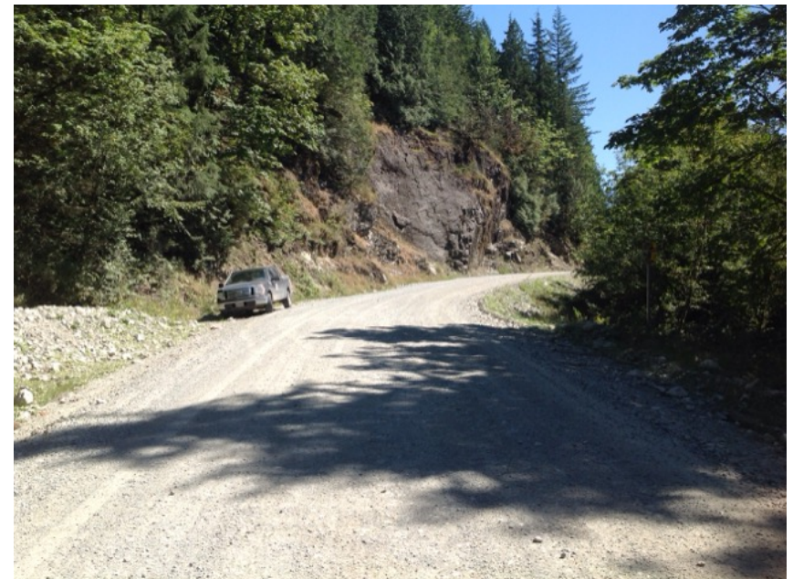
Approach from Right Bank when facing downstream
